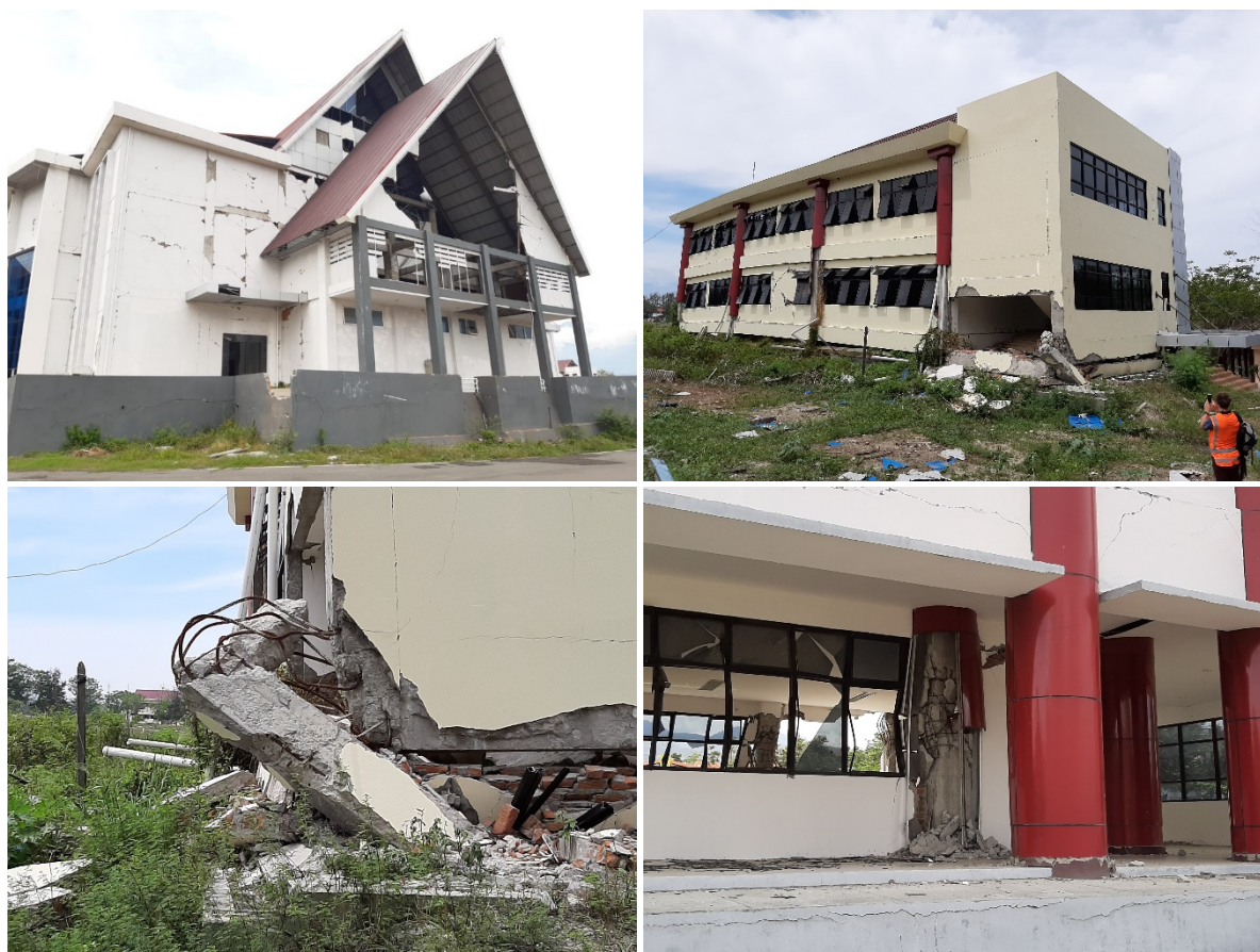
Figure 2: Field observations at Universitas Tadulako. Auditorium with out-of-plane failure of large unreinforced masonry gable (top left), Faculty of Forestry with complete collapse of ground floor (top right), Faculty of Forestry joint shear failure (bottom left), and Faculty of Law ground floor column shear failure (bottom right).
