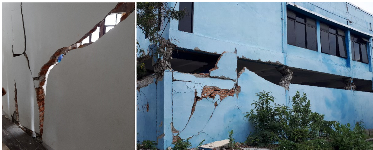
Figure 3: Field observations of government buildings. Large crack in a masonry partition wall crossing a seismic joint in the Palu City Mayor’s Office (left), and failure of ‘short’ columns in the Main Palu Fire Station (right).
