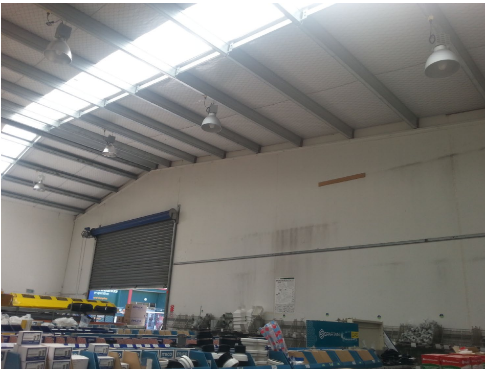
Figure 3: View from inside of Grid 1 wall
