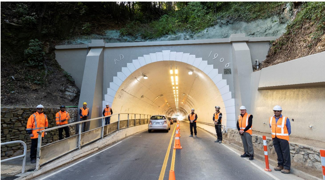
Figure 7: The proud project team at the Strathmore portal end after completion.
