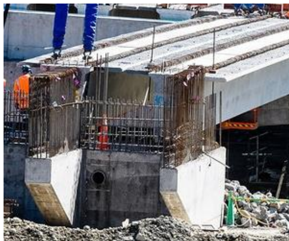
Figure 3: Super-t girder 'stability tie' system is very efficient while providing enhanced robustness over conventional girder bracing strategies.
