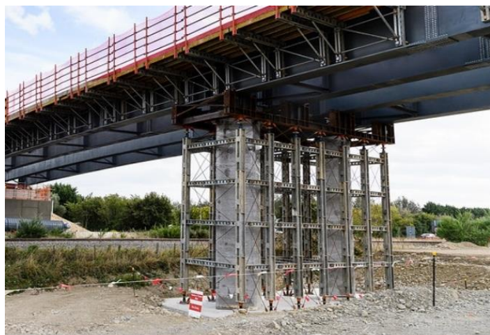
Figure 4: Bridge BR08 propping at Peka Peka to Ōtaki showing ‘composite’ temporary/ permanent load path. Photo credit: Mark Coote.
