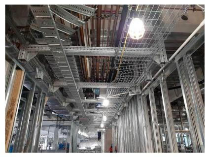
Photograph 6- View of frame in congested corridor area while services installation is occurring Paper 146 – Wellington Children's Hospital- a different approach to a seismic restraint project
