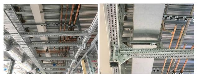
Photographs 1 and 2- Cradle frames with installation of services occurring
