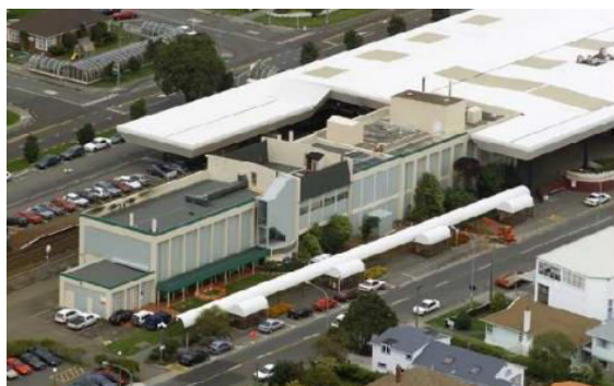
Figure 1: Waterloo WTP aerial view.
