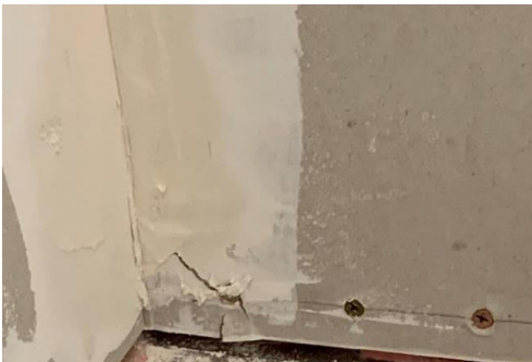
Figure 6. Significant local plasterboard damage in east and west walls
