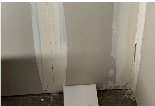
Figure 7. Opening of vertical plasterboard sheet joints
