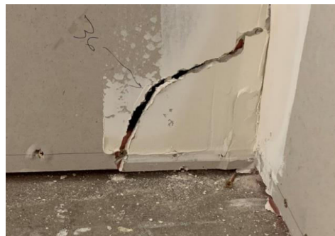
Figure 6. Significant local plasterboard damage in east and west walls
