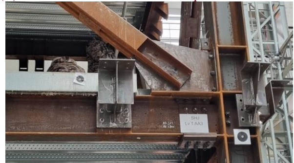
(c) Sliding Connection at Brace Bottom Before SHJ bolts removed
