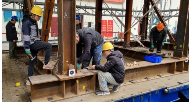
(b) Fixing Column Base Connection (1)
