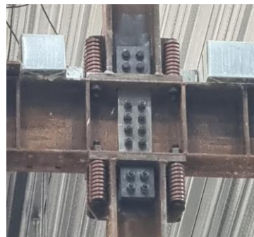
(c) Rocking Column Detail
