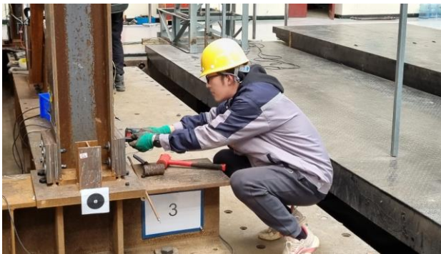
(c) Fixing Column Base Connection (2)
