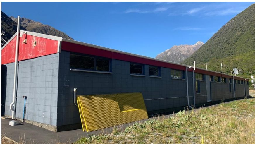
Figure 3: Example of typology 3 building
