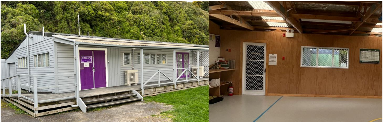
Figure 1: Example of typology 1 building
