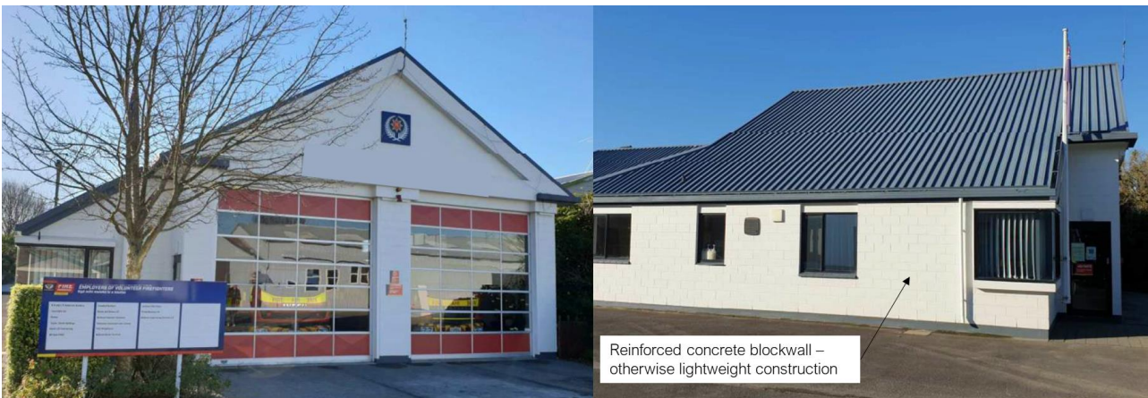
Figure 2: Example of typology 2 building
