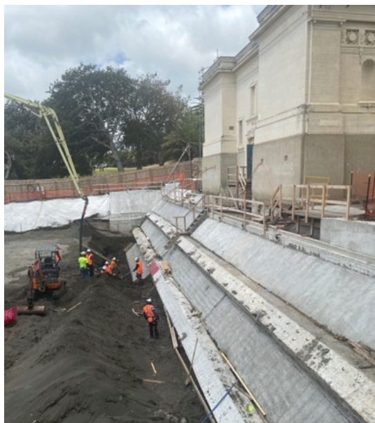
Figure 12: Temporary anchored wall to support the adjacent basement excavation
