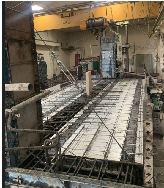
Figure 3: Specimen before concrete pouring
