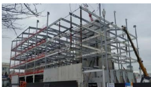
(a) A five-storey commercial building with steel gravity frames, core and perimeter concrete walls, and an internal eccentrically-braced frame. Photo: Bruneau and MacRae (2017)
