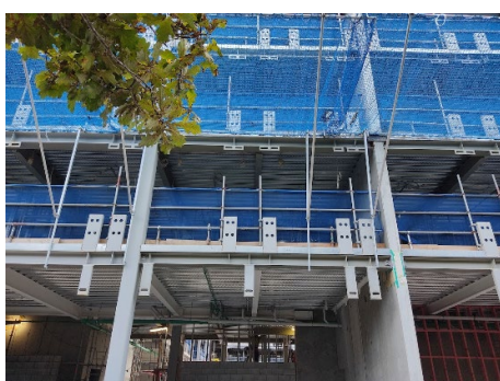
(c) A nine-storey apartment building in Auckland with concrete walls and steel gravity frames.
