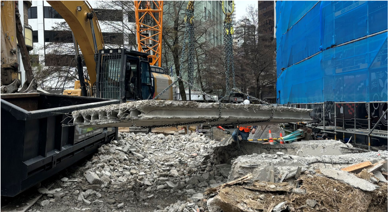
Figure 19: Chance view of hollowcore web splitting during demolition removal, 13 Sept 2024
