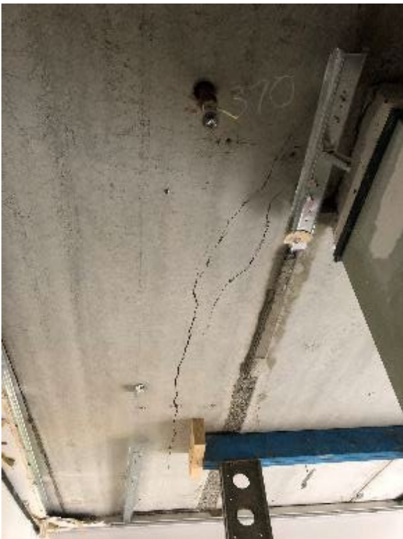
Figure 18: Photo from the Aurecon L2 soffit mapping adjacent northern stair void (grid 27)
