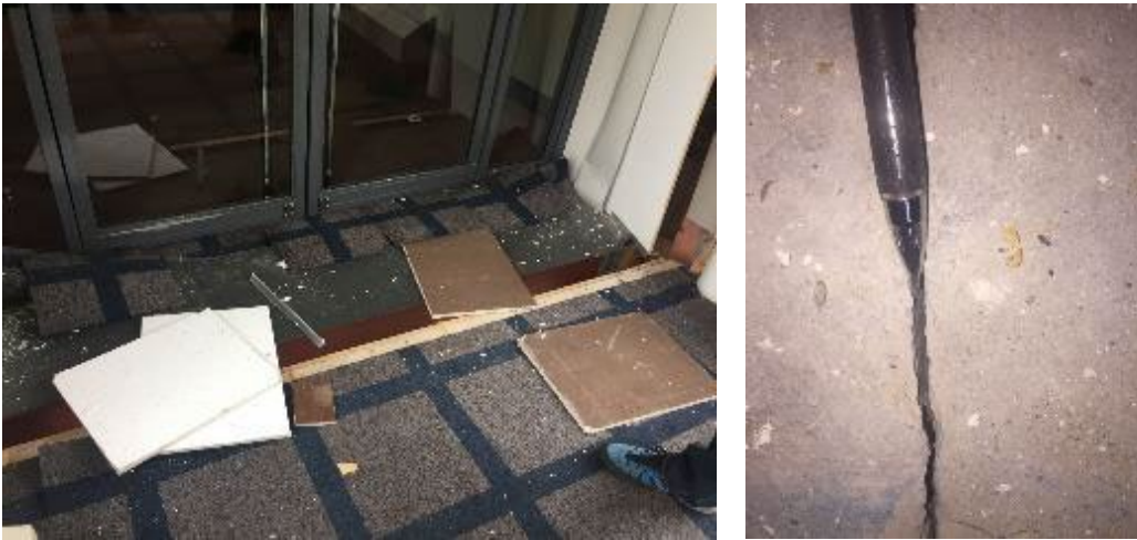
Figures 4-9: A selection of photos taken during rapid building inspection(s)
