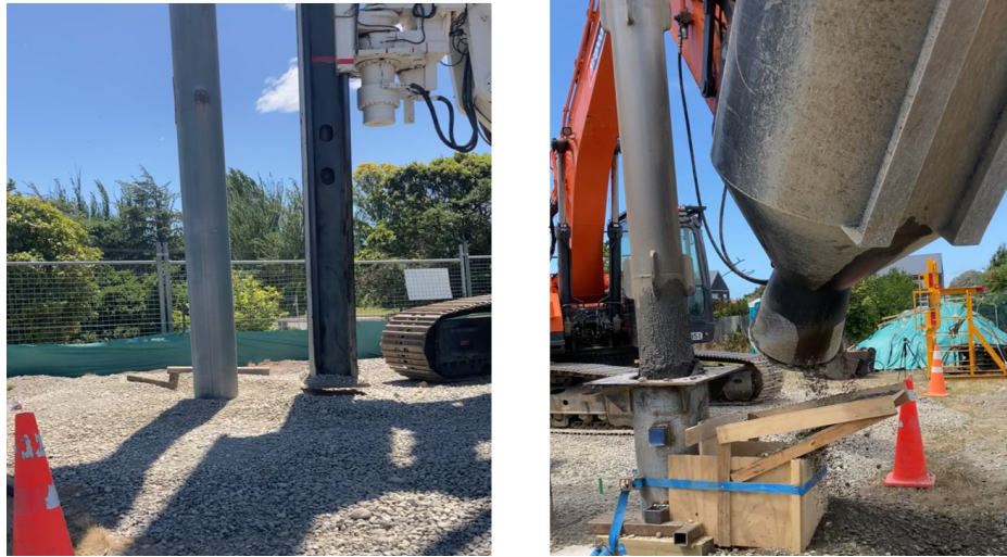
Figure 3: Rig working on a 300 mm gravel pad, showing (left) the casing and mandrel set being lowered and (right) a hopper feeding aggregate (right) at the Wainoni SCRR pilot project site.
