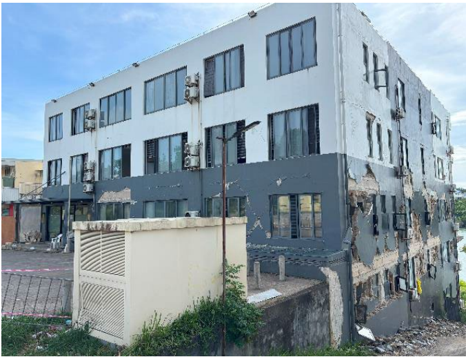
Figure 18 and Figure 19. Major damage to masonry walls on side of building, minor-to-major damage at front. Concrete frame appeared to be generally intact. Close up of damage.
