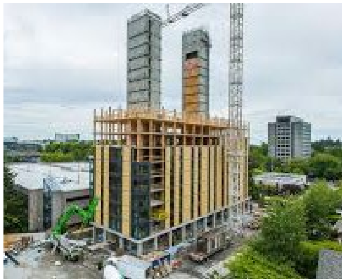
Figure 1: Timber building with concrete cores.
