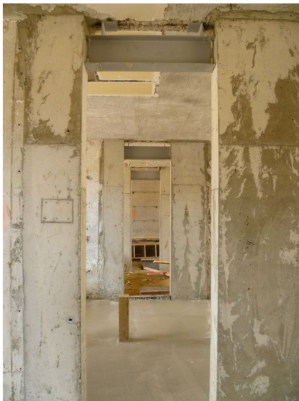
Figure 2 Newtown Park Flats, examples of de-stiffened walls and modifications to coupled walls from (Cattanach 2013)
