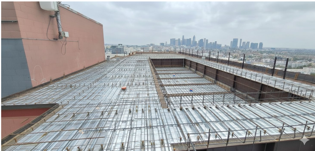
Figure 1. Roof Top Pool Deck and Hot Tub
