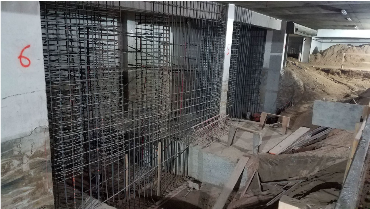
Figure 3. Progress Photo of New Shear Wall – Existing Wall Interaction at Foundation Level Construction
