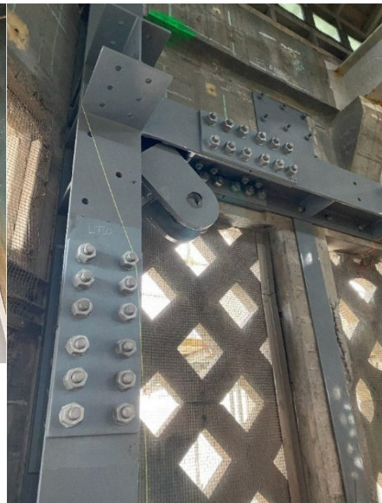
Figure 9: Steel portal frame at Level 8 and double cleat for the viscous damper install.
