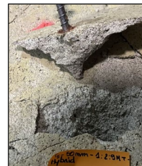
(c) Tension test - Cone failure
