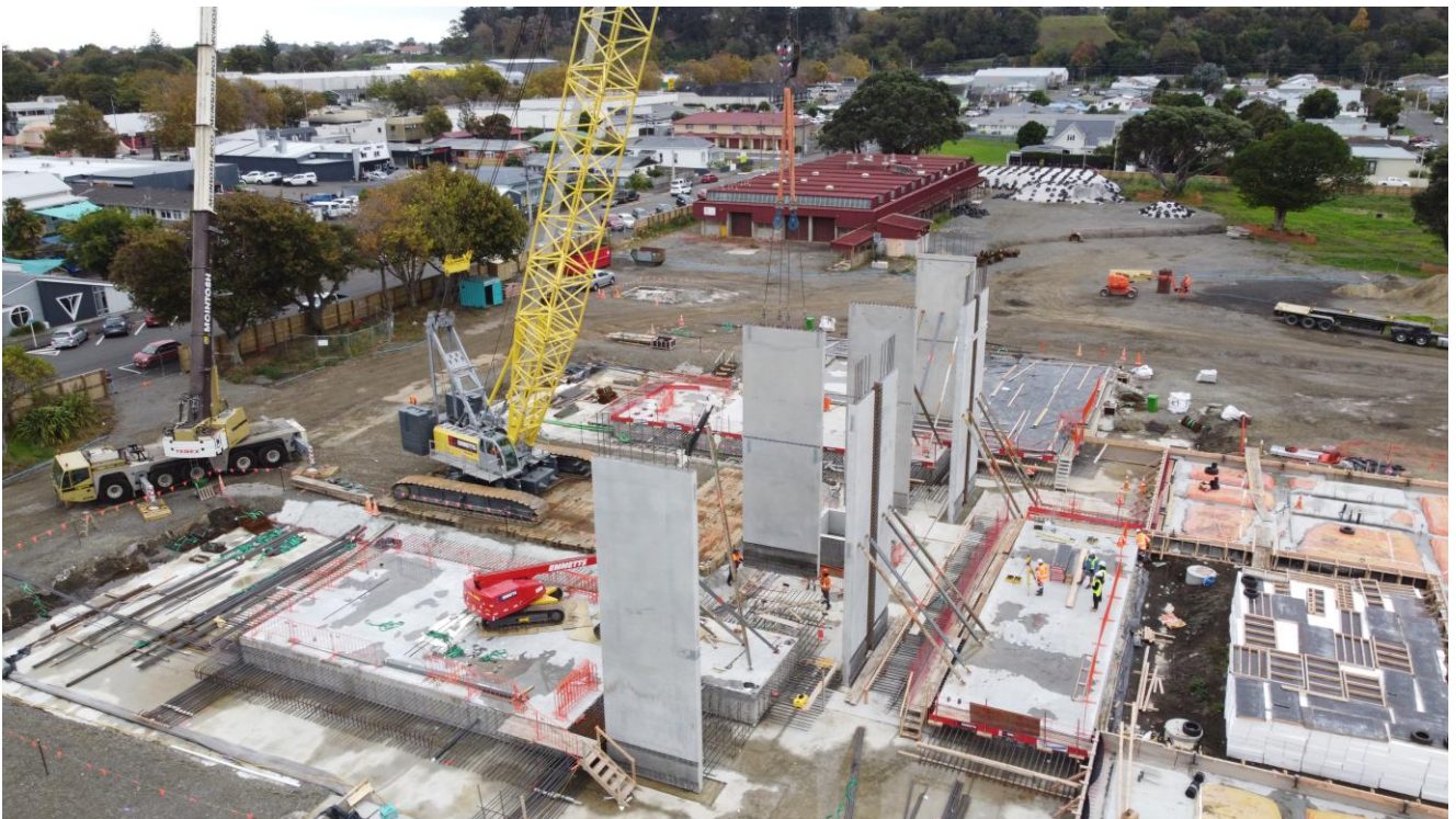
Figure 7: Precast shear wall installation in progress
