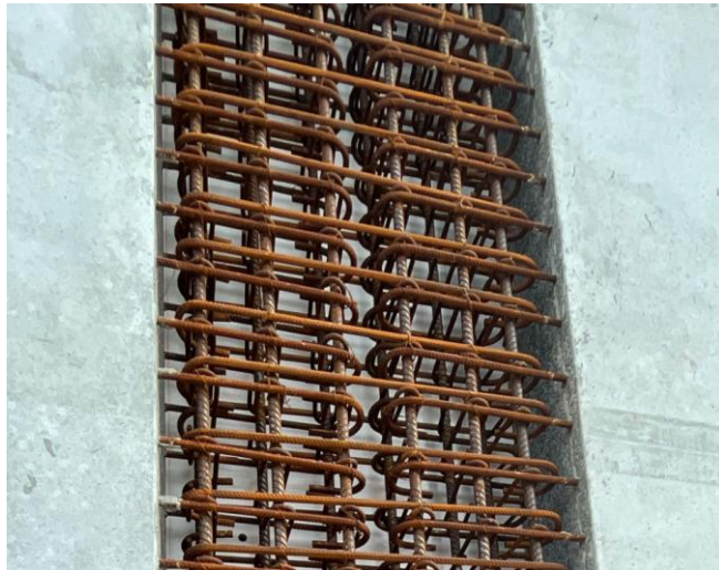
Figure 6: In situ stitch joint construction example
