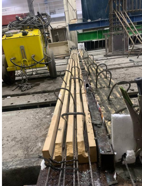
b) Ribs During Groove Grouting
