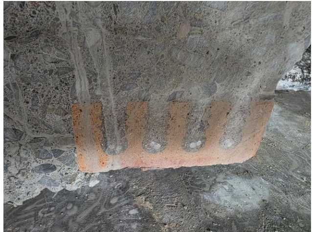
b) Close-up view of the rib section
