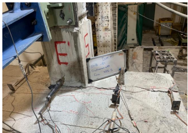
f) Beam–Slab Interface Crack at 4% Drift (East Side)
