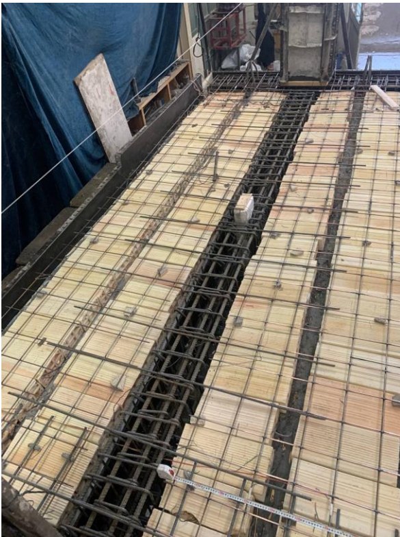
c) Specimen Prior to Concrete Pouring
