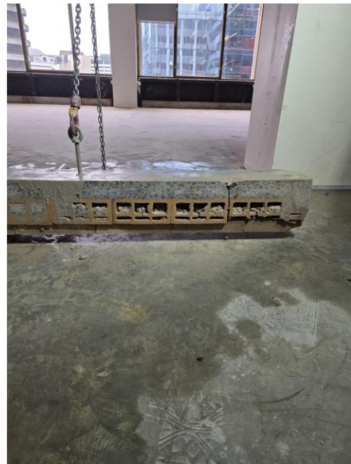
c) Close-up view of the hollow-block infill section
