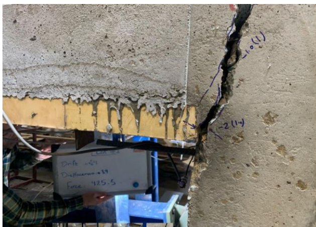
e) Negative Moment Failure at Rib Ends (East Side)
