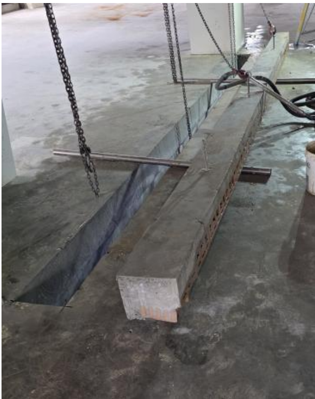
a) Extracted prestressed rib
