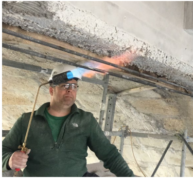
Figure 13: Flexural strengthening of bridge girders and deck soffits
