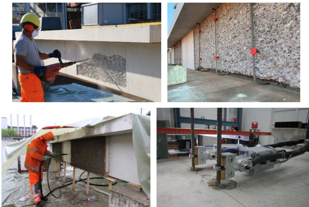
Figure 9: Surface roughening, rebar installation, sprayed mortar application, resistive heating, (Czaderski et al. 2019)
