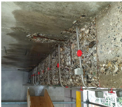
Figure 14: Shear strengthening of bridge girders
