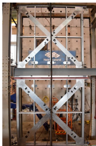
(f) Test 3 (before test)
