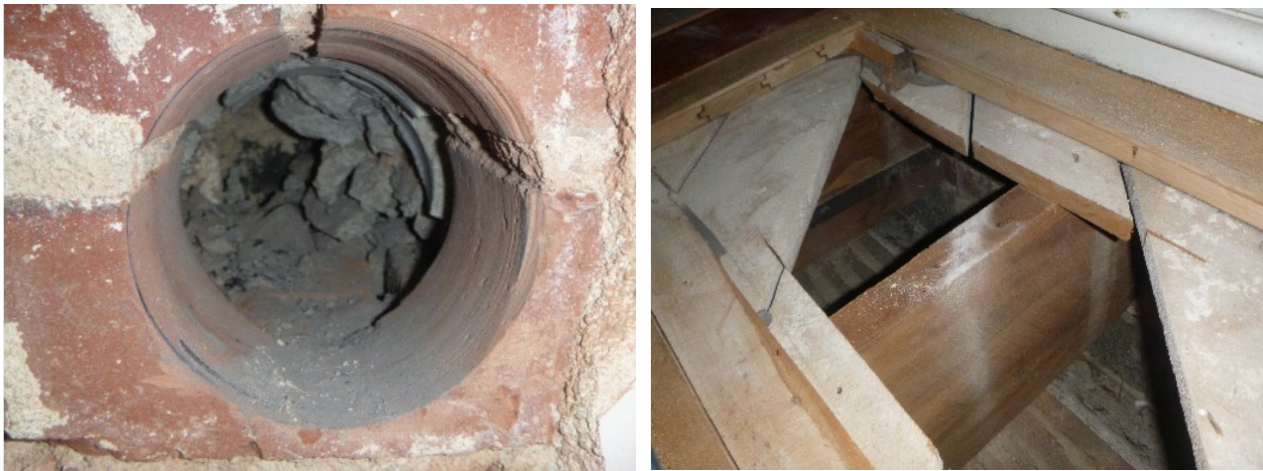
Figure 3: Sample photos of intrusive investigations
