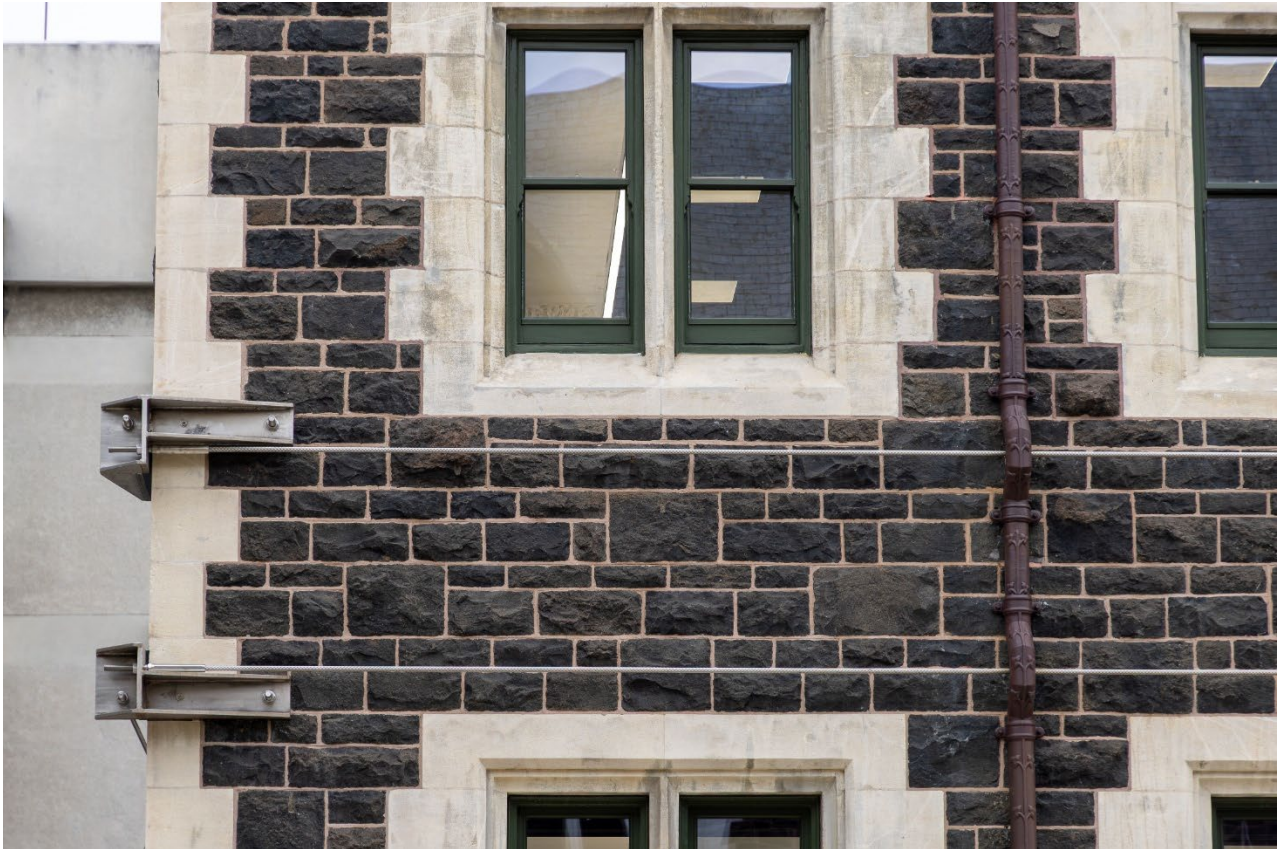
Figure 5: External post-tensioning brackets and cables (Credit: Cook Brothers Construction, University of Otago)
