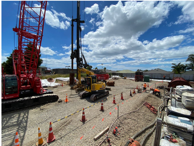
Figure 5: Bored piles being constructed by March Construction
