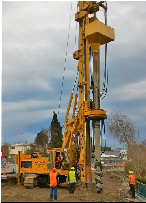
Figure 3: McMillan Civil's non-vibratory stone column rig
