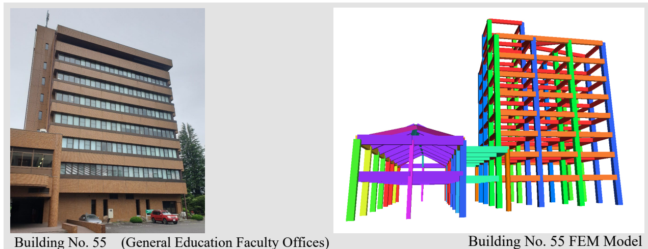
Figure 2: Exterior views and FEM model of Buildings No. 55
