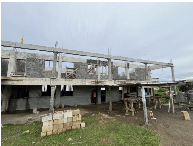
Figure 5: Concrete frame with masonry infill typology (Left), Observed URM infill failures (Right)
