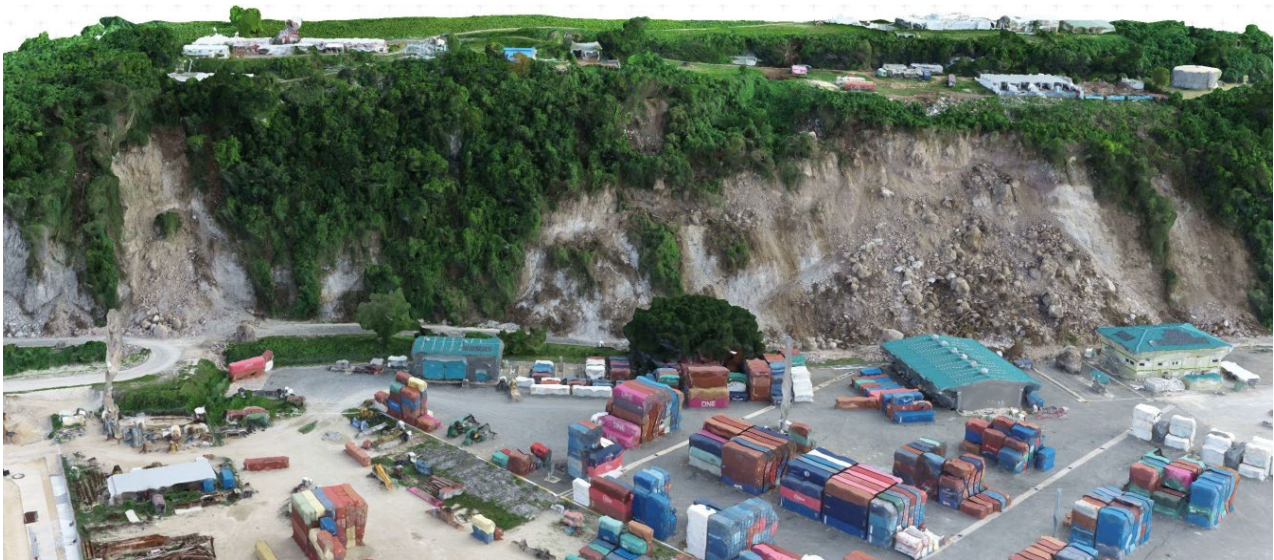
Figure 1: Wharf Road Landslide
