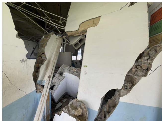
Figure 5: Concrete frame with masonry infill typology (Left), Observed URM infill failures (Right)
