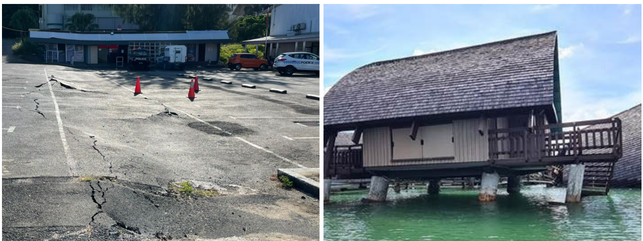
Figure 3: Ground damage effects at Port Vila CBD (Left), Erakor Lagoon (right)
